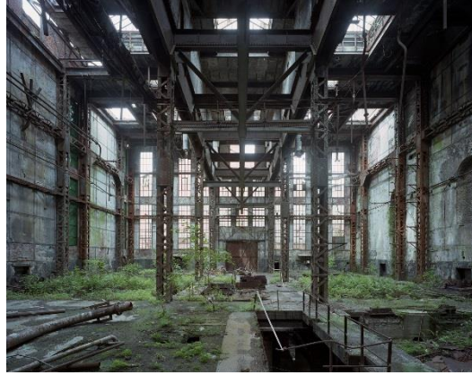
Figure 1.3 Boiler Room, Argentine. Yves Marchand et Romain Meffre, 2014.
