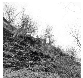
Figure 1: Photos du site
